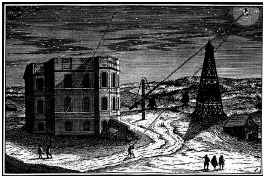
Fig. 3 A woodcut showing observers in the foreground, in front of the Paris Observatory, using two of the very long focal length refractors. Their objectives were attached to the Observatory building itself (in the case of the left-hand pair of observers) and to the Marly Tower (in the case of the right-hand observer). The eyepieces of these telescopes were held by the observers. The lines apparently joining the objectives and the eyepieces in this woodcut are there to indicate the incoming light rays, not tubes, as these telescopes lacked tubes (indeed these were referred to as ‘telescopes without tubes’ by Cassini). Meanwhile, the much shorter focal length telescope in the background, on the terrace and attached to the mast, does have a tube (After Wolf 1902)
